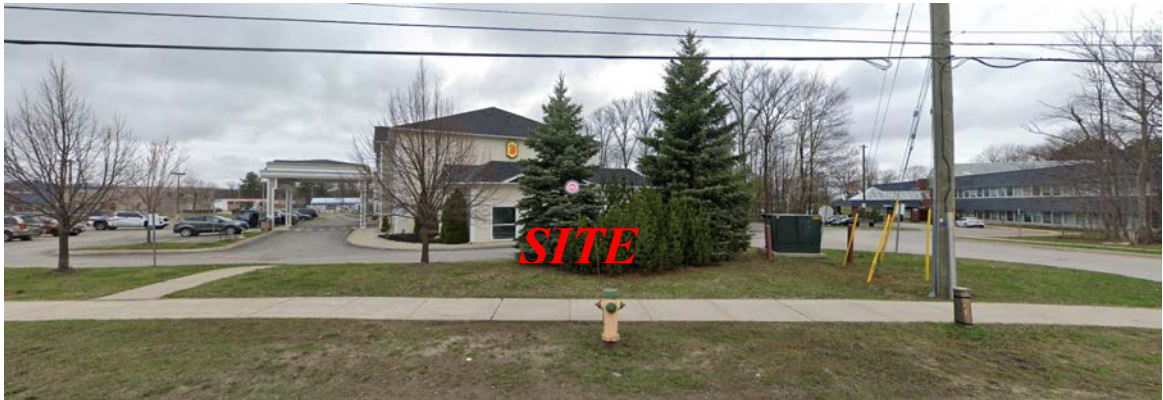
Figure 2 - Site Existing Condition
