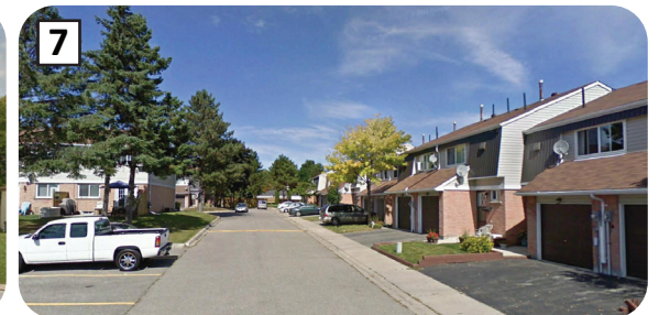
Existing condominium townhouse development
