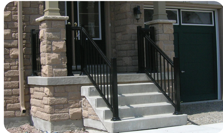
Masonry Porch with Precast Steps
