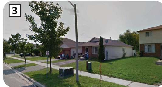
Existing homes on Frazer Dr.
