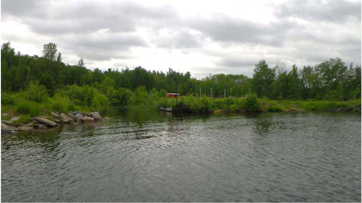
Photo 19: Embayment and Collapsed deck and light standard, Centre Reach
