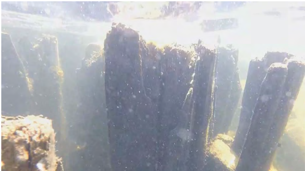
Photo 14: Timber piles at west end of East Reach (Day 1, Dive 1, 1:33:37)
