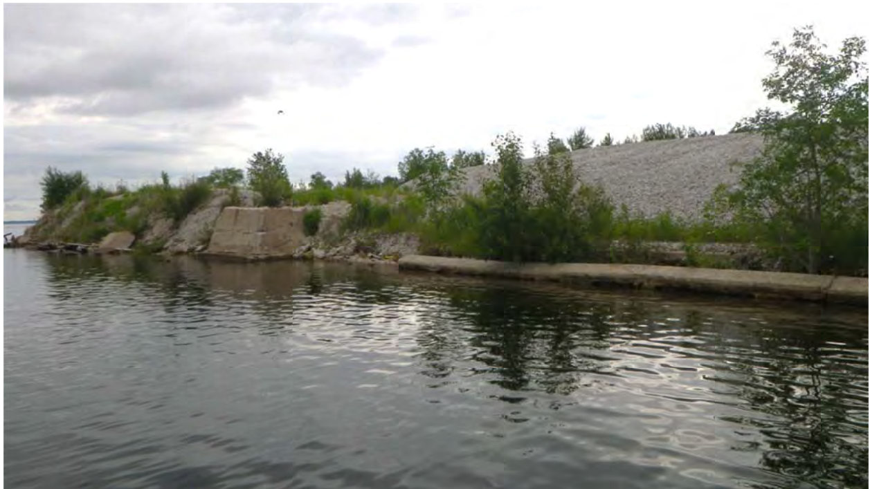
Photo 26: Large concrete foundation in east part of West Reach
