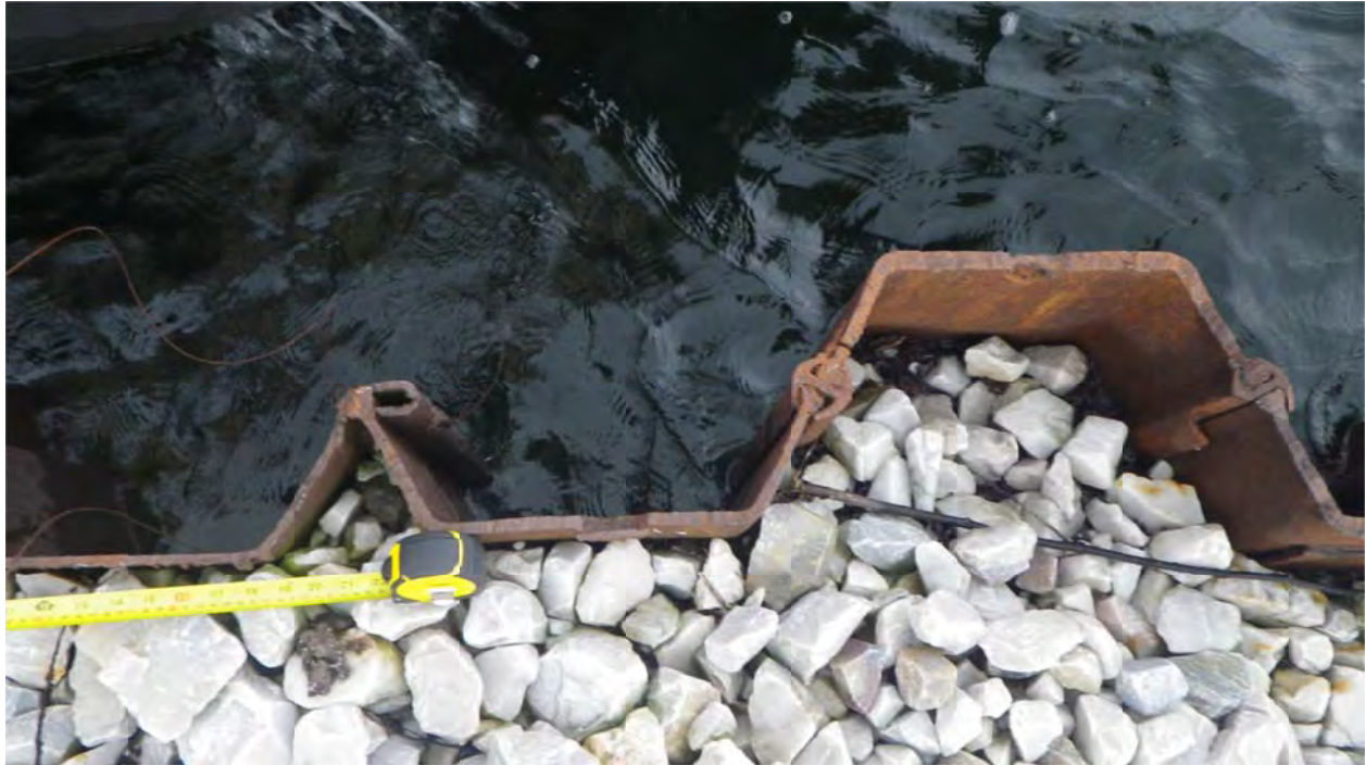
Photo 31: Interface between U-series and Algoma SSP wall, West Reach
