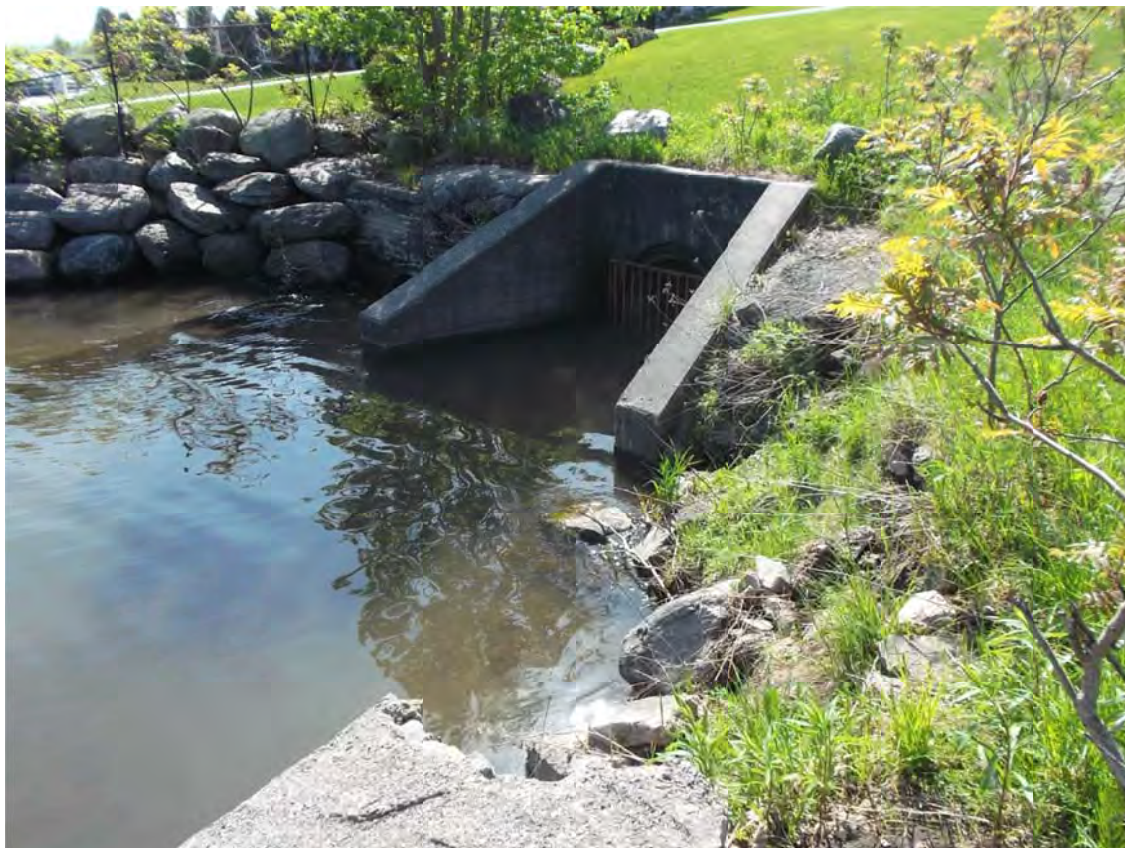
Photo 34: Outfall at east end of property
