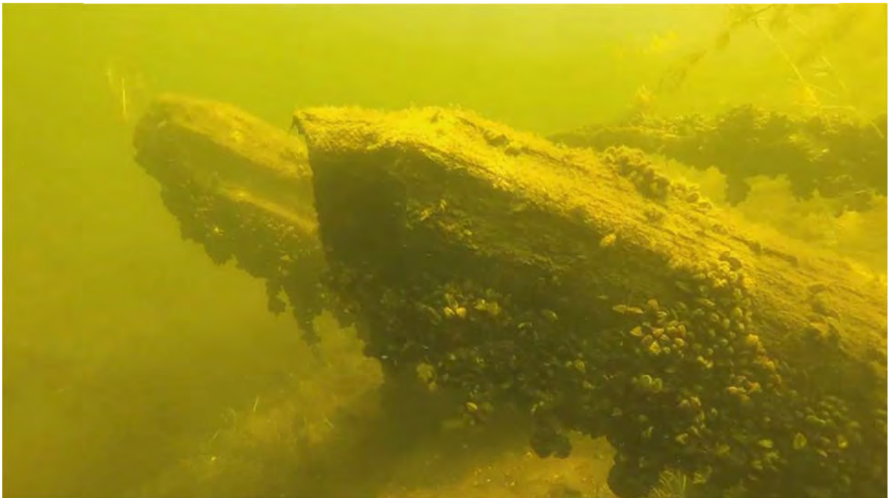
Photo 16: Timber Piles in Centre Reach (Day 1, Dive 1, 1:49:37)
