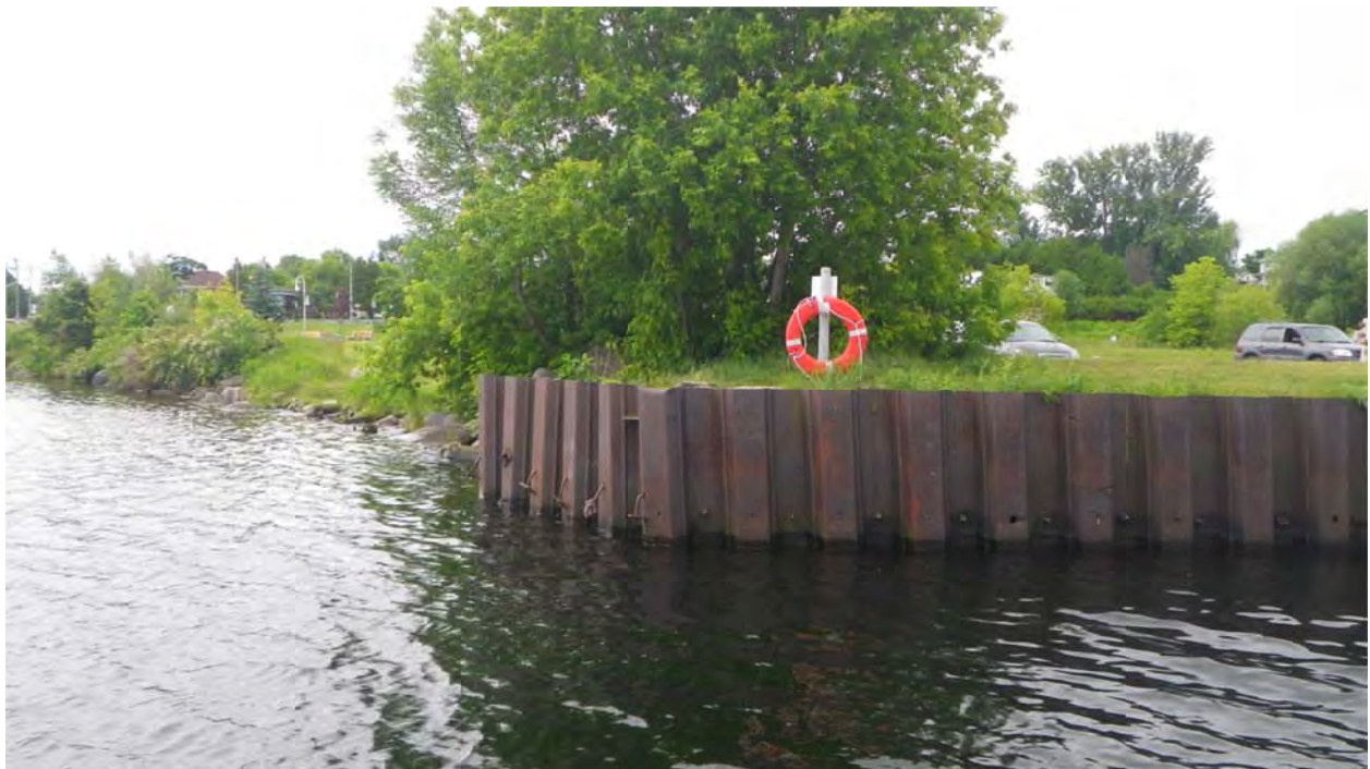
Photo 32: East end of SSP wall, East Reach
