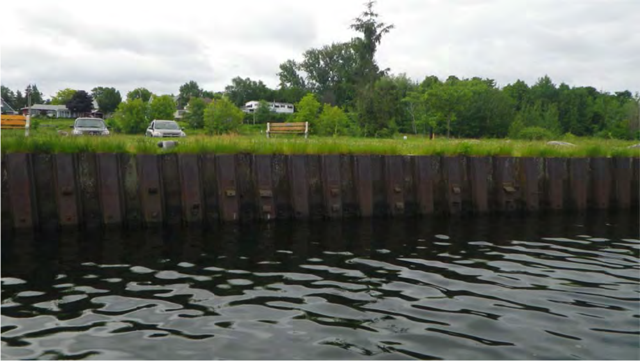
Photo 2: SSP Wall, East Reach
