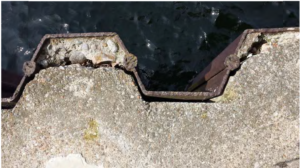
Photo 6: SSP separated from concrete relieving platform, East Reach
