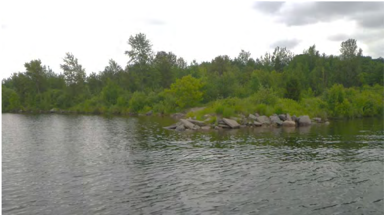
Photo 18: Concrete rubble and armour stone headland in Centre Reach
