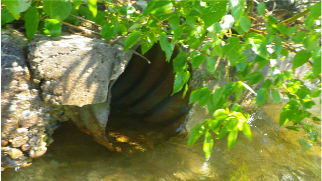
Photo 29: Corrugated Steel Pipe in West Reach
