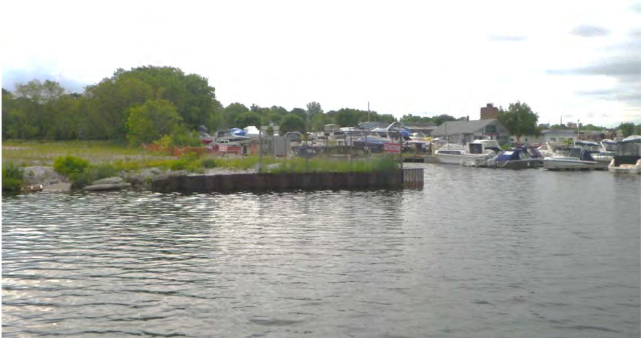
Photo 30: SSP wall at west end of site, West Reach
