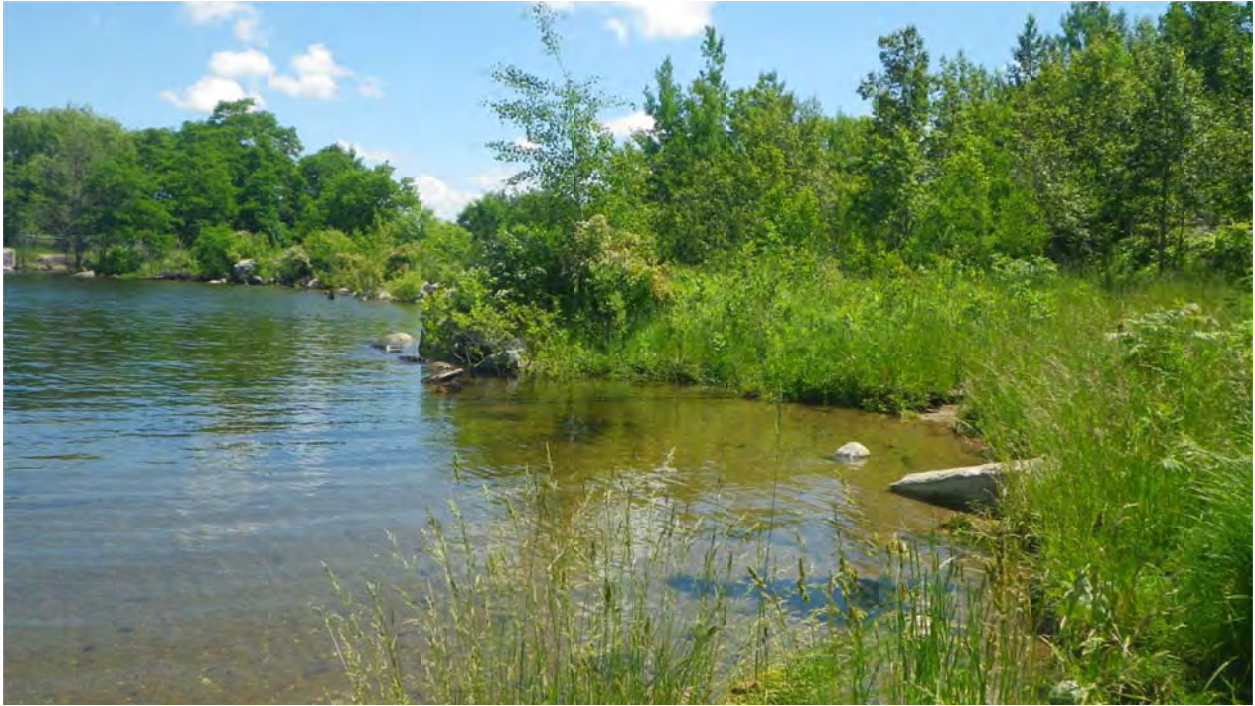
Photo 11: Shoreline behind collapsed SSP wall, East Reach
